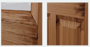
In an unsealed wood door, water seeps in around the glass and panels, which can lead to damage in the form of cracking, splitting, delamination, bowing or warping of your wood door.
